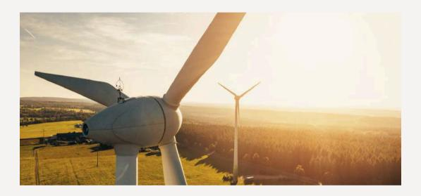
Wind projects are often located in remote areas with limited infrastructure, increasing the risk of access delays, weather disruption and labour shortages. Transporting large components like blades and nacelles (the top sections of wind turbines that contains the gearbox, generator and control systems) requires upgraded roads and precise logistics coordination, which can affect civil works.
